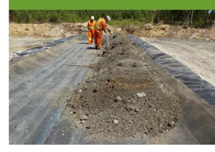
**Treatment:** The soil cell was built at the client site and divided into sub-cells. Soil type varied. The picture above shows the initial construction of the soil cell.
